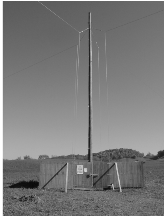
Figure 5 - Kinstar antenna center section and support pole.
